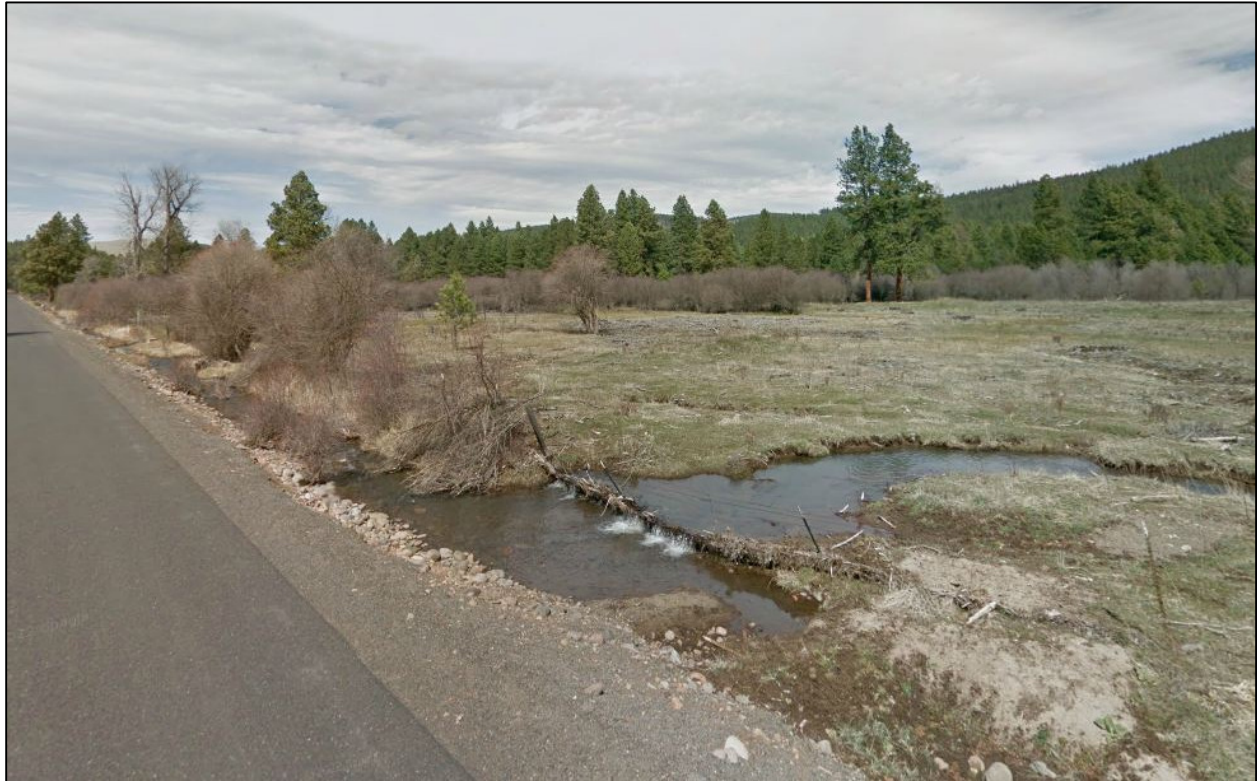
Side channel and bar ditch confluence on OR 203 near OSU's Hall Ranch
