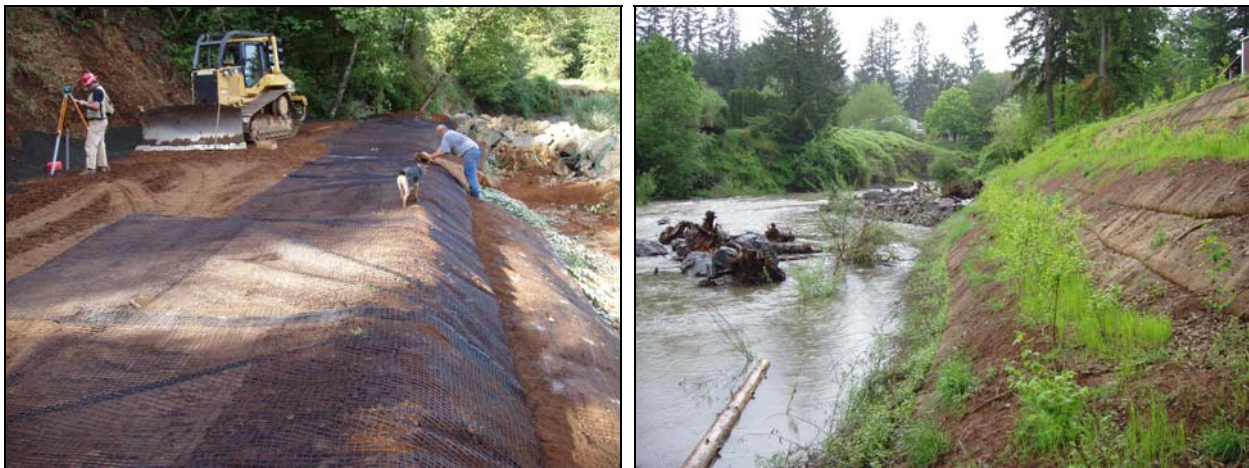
Figure 4. Example of engineered soil lift used for bank stabilization and vegetation growth.
