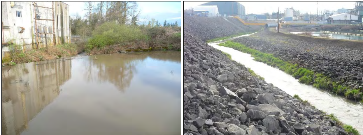
Figure 4-36. The concrete dam on lower Cox Creek is a fish passage barrier to upstream migration (left). Truax Creek was formerly used to dispose of industrial wastes. Contaminants were removed from the stream corridor and the creek was stabilized (right). Treated wastewater from the ATI-Wah Chang facility is discharged to Truax Creek, providing flow in lower Truax Creek after the upstream seasonal stream dewateres in the summer.
