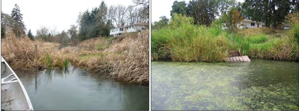
Figure 4-29. The outlet at West Thornton Lake at moderate flows in January 2011 when the natural outlet was overtopped (left) and during summer conditions when the lake level is below the outlet elevation (right). A board is placed in the culvert inlet to block outflow from the lake. The culvert allows for drawing down the lake an additional 1-2 ft below the outlet.
