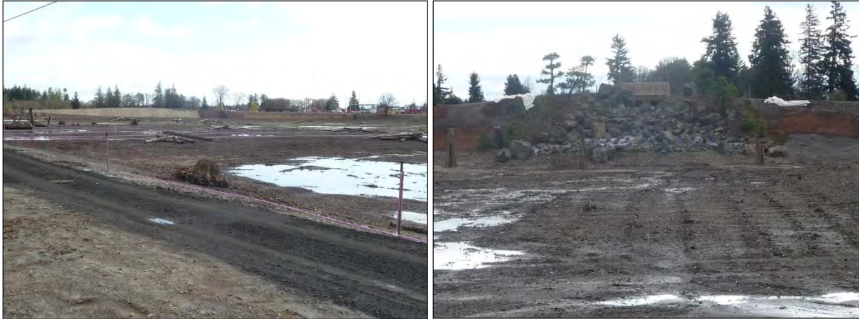
Figure 4-39. A view to the northeast across the Talking Water Gardens wetlands (left) and a view of one of the five aeration waterfalls planned for the site (right). The treatment wetlands will provide recreational and educational opportunities for the local community as well as cool and remove nutrients from treated wastewater.
