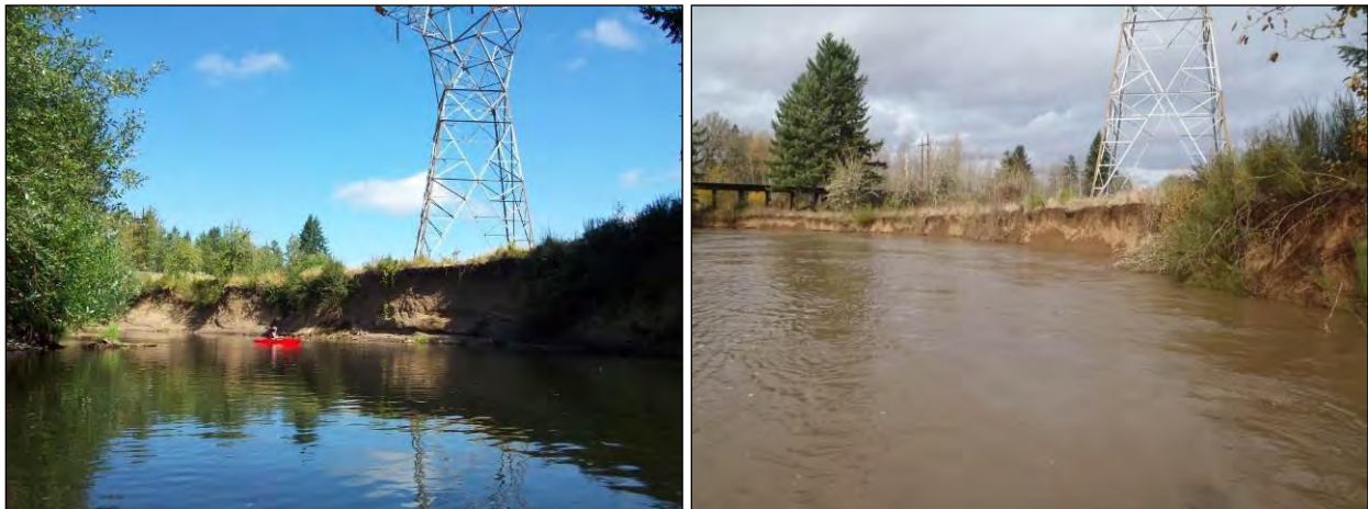
Figure 3-9. A comparison of river conditions associated with low (left) and moderate (right) flows on the Calapooia River downstream from SW Queen Avenue Bridge. The height of the eroding bank is masked by moderate flows but the magnitude was apparent during the summer field data collection.
