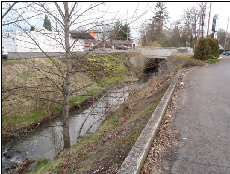
Figure 3-10. Periwinkle Creek downstream from the SE 9 th Avenue Bridge. This reach marks the start of the more urbanized reach of Periwinkle Creek. The riparian zone has been narrowed to a fringe and impervious surfaces such as roads and parking lots accelerate stormwater discharge to the creek. Stream corridor modifications have allowed development to expand to the stream edge while protecting against flooding.
